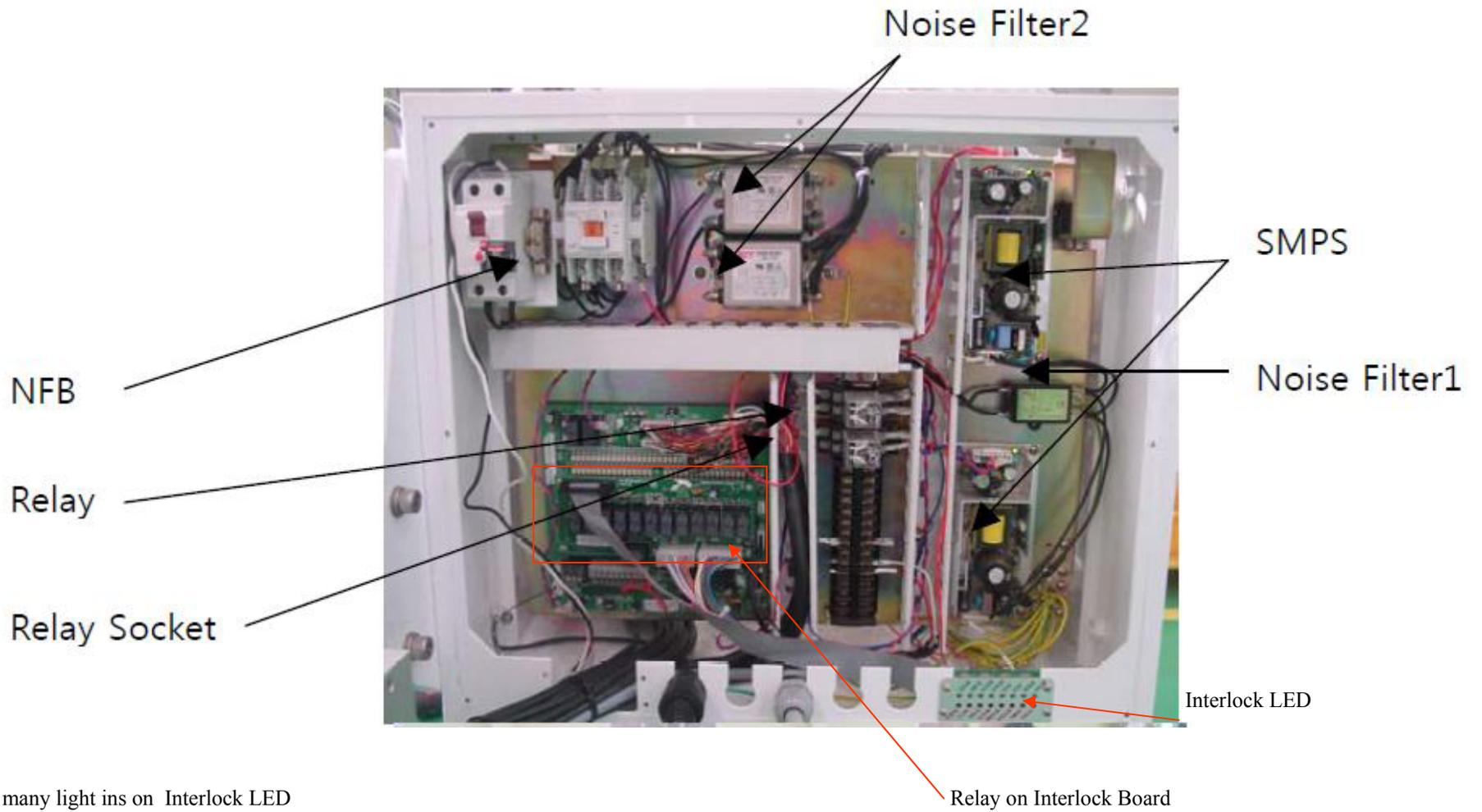
1. Check how many light ins on Interlock LED
